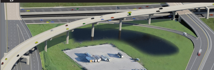
Figure 6 - Piers in Pond H-6
