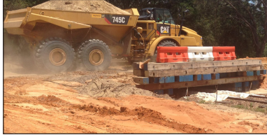
Figure 20 - Air Bridge over FGT
